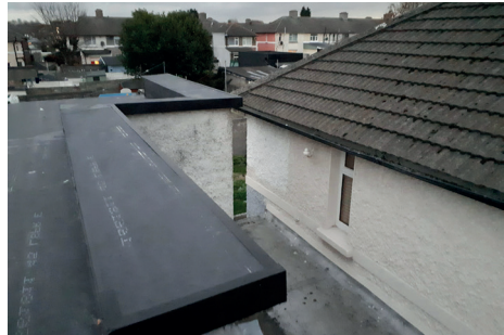
Example of Flat Roof External Insulation
