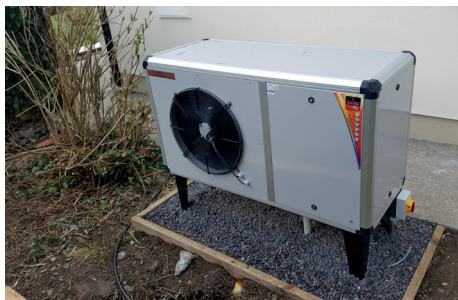
Example of external unit of an Air to Water Heat Pump
