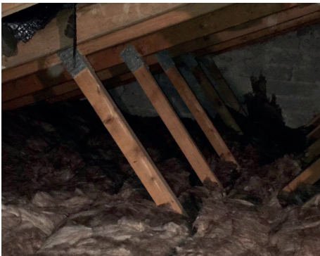
Rockwool insulation rolled out in attic
