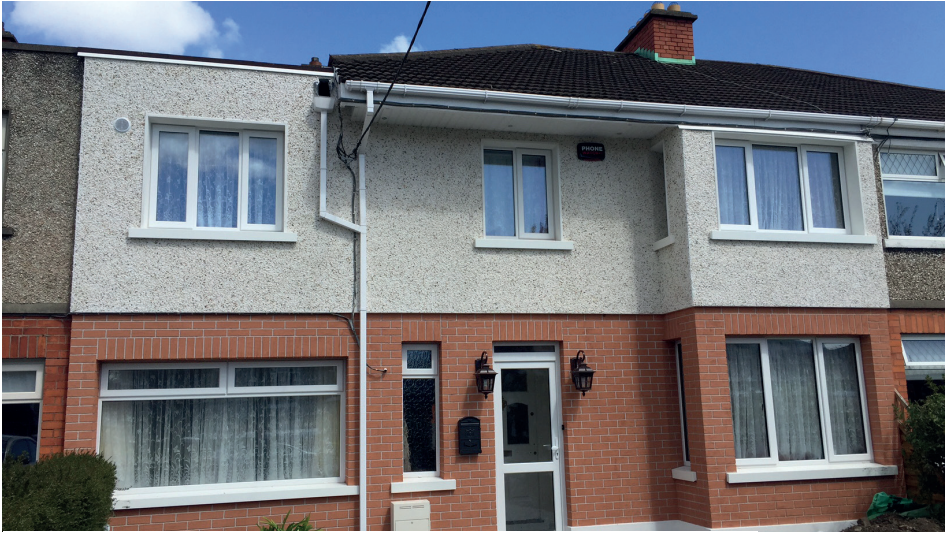
Example of External Wall Insulation with pebble-dash
