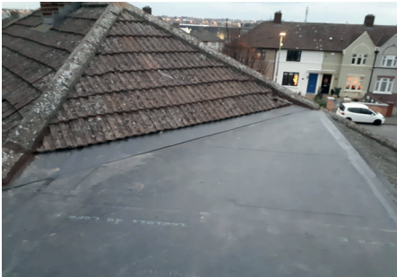
Example of Flat Roof External Insulation
